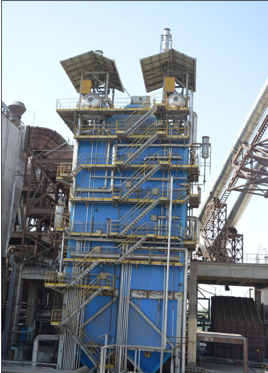
Waste heat recovery Power generating Boiler Unit
